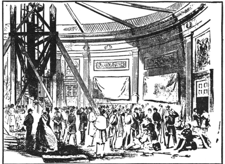
Living quarters for the Eighth Massachusetts Regiment in 1861 were found in the unfinished rotunda of the Capitol Building.
